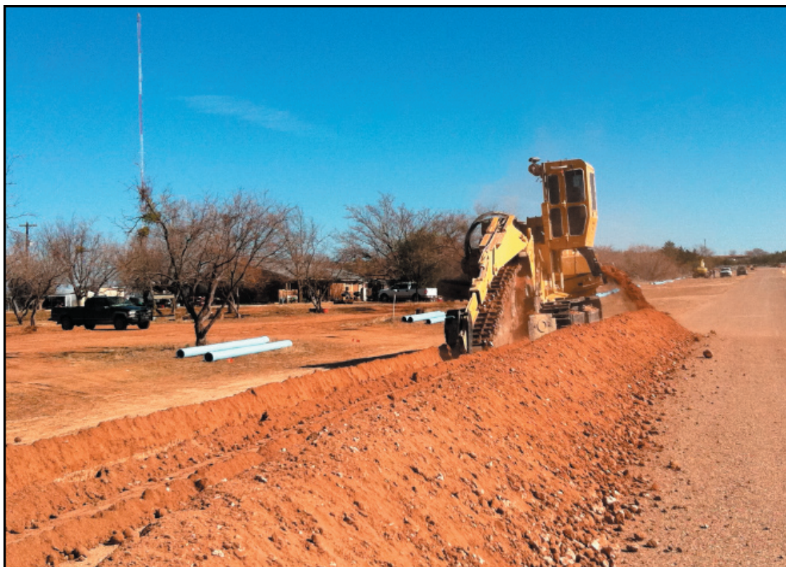
It's Begun! The trench for the water pipeline is under construction. Digging began Tuesday, with the machine and its operator being donated by Vermeer.
