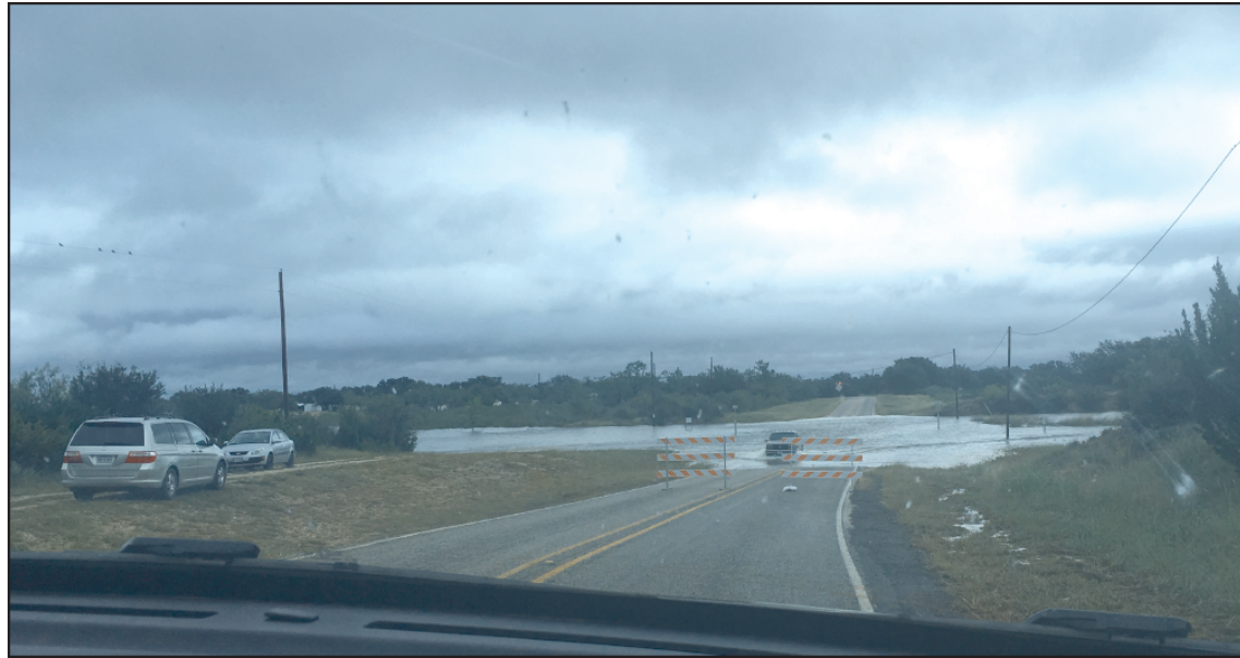
High Water! Residents who have to travel Lake Dam Road at Oak Creek Reservoir are encountering major difficulties in accessing their homes. TxDOT closed the road at the spillway west of the dam. High profile vehicles appear to be able to cross the spillway. However with abundant rain this past week, other low water crossings either are or may become impassable. Residents in many Texas areas have experienced severe flooding in the last week or so. Remember, turn around - don't drown!
