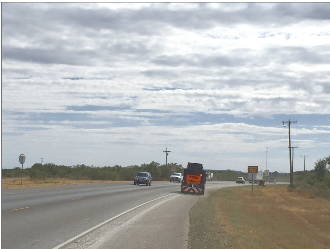
Highway Safety! TxDOT crews were out in force Monday, October 5, 2015, adding safety features in the four miles of US Highway 277 just north of Bronte. They first brought in a radar trailer a couple of weeks ago and this week, they cut in rumble strips. The strips run just outside of the white lines and down the center of the highway.
