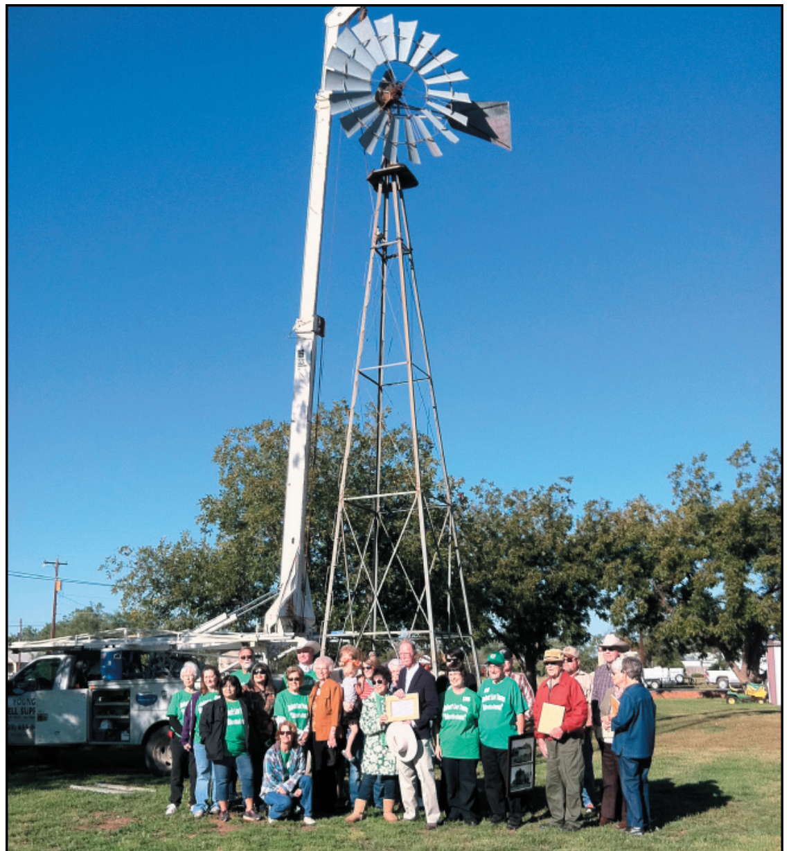
Windmill is Up! Members of Robert Lee Vision with a Purpose were on hand Tuesday morning as the windmill, donated by Ed Blackburn, was erected on the Coke County Courthouse lawn. It is one of the first additions to the new Coke County Memorial Garden. This project, sponsored by Robert Lee Vision with a Purpose, will have paving stones available for purchase. These stones are the perfect way to honor or memorialize a person or event. Order forms are available at Coke County Library, Robert Lee City Hall, Coke County Courthouse or B's Blossoms N Bloom. In addition to Mr. Blackburn donation of the windmill, Young Well Supply donated the time and equipment used to erect the windmill.
