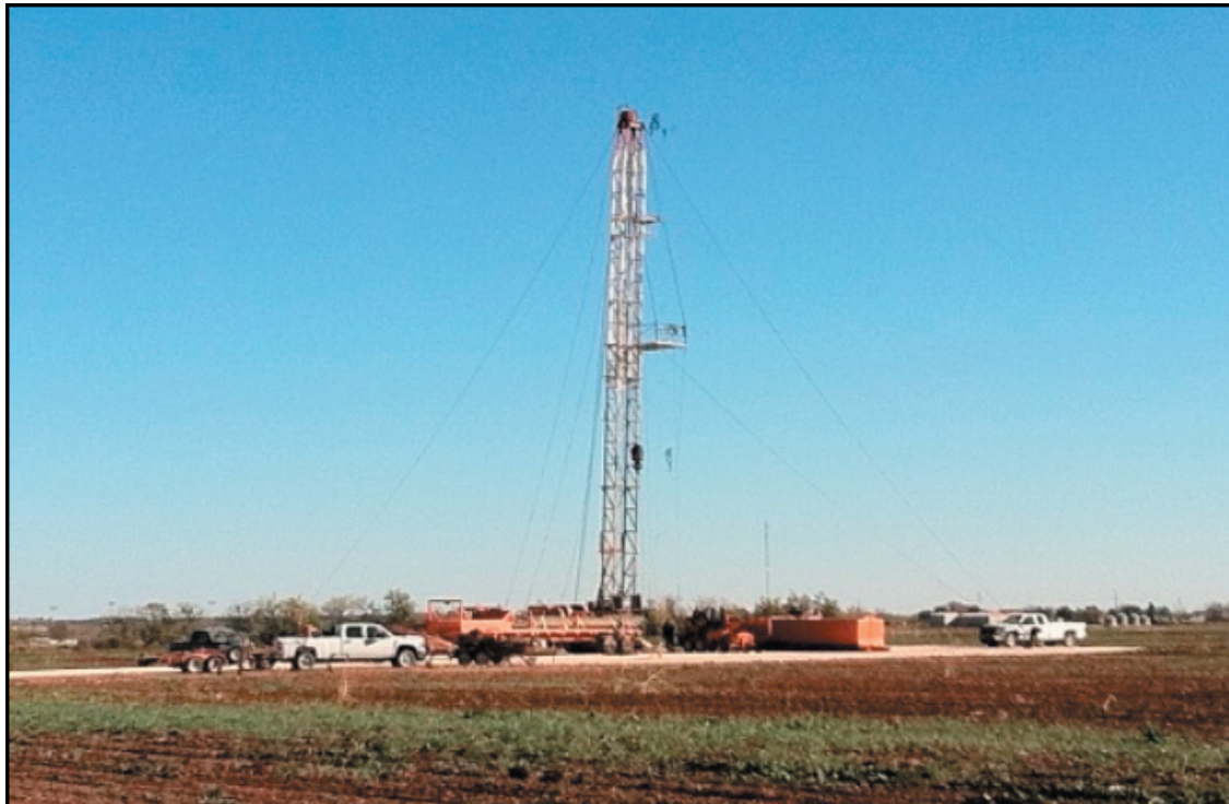
Oil Boom Coming?! Many rumors have been floating around Coke County that the Oil Boom is Coming! These rumors may or may not have some truth to them, but following the seismic testing along Hwy 158 between Bronte and Robert Lee, this workover rig was erected this week about a mile west of Bronte on the south side of Hwy 158. Due to recent technological advances, old wells are being retapped to capture oil that old technology could not recover.
