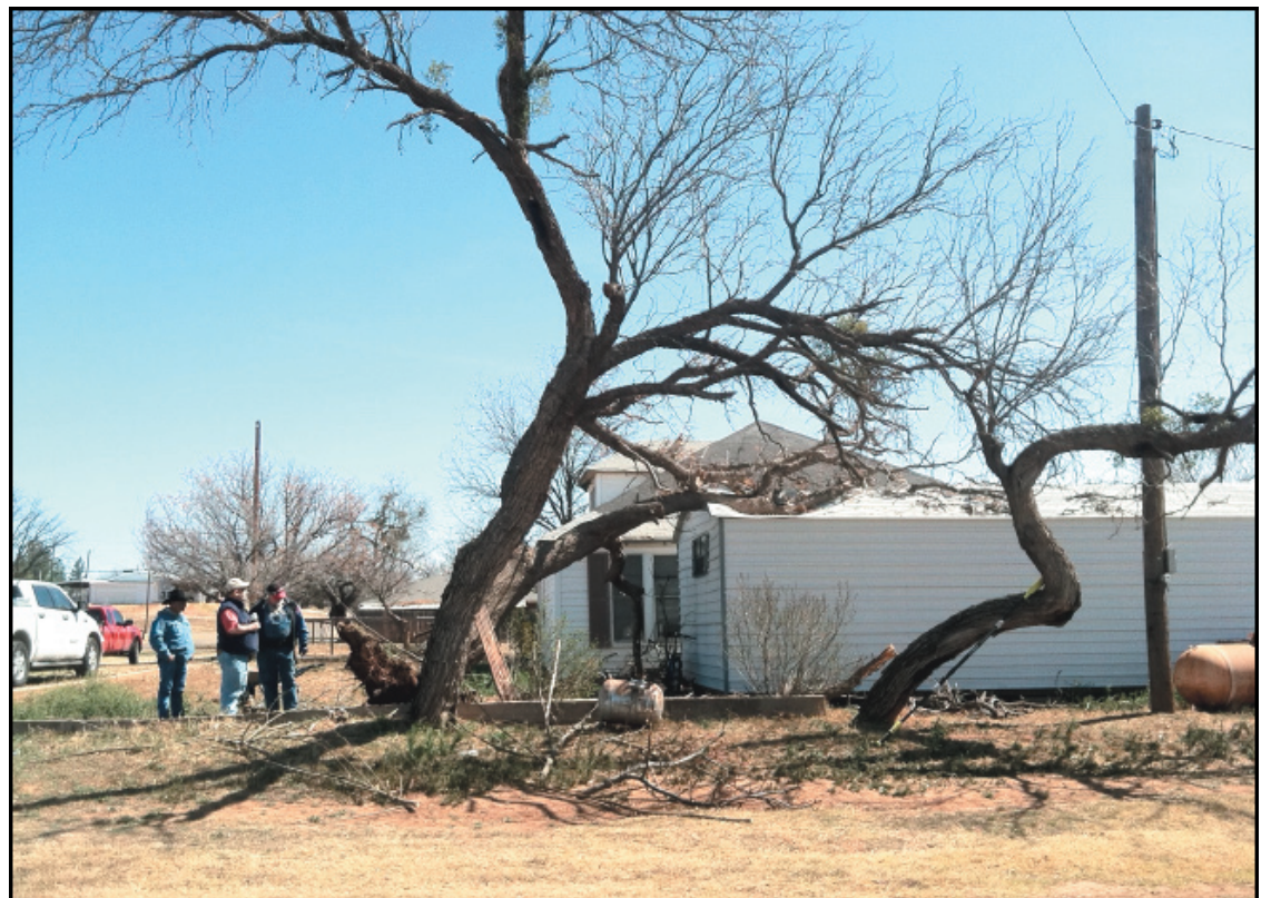
Storm Damage! This huge tree fell Monday night on the home of Leroy and Jami Casey across from the football field in Robert Lee during the awful windstorm. The damage included the building in the front of the photo and also portions of the home's roof behind the building.
