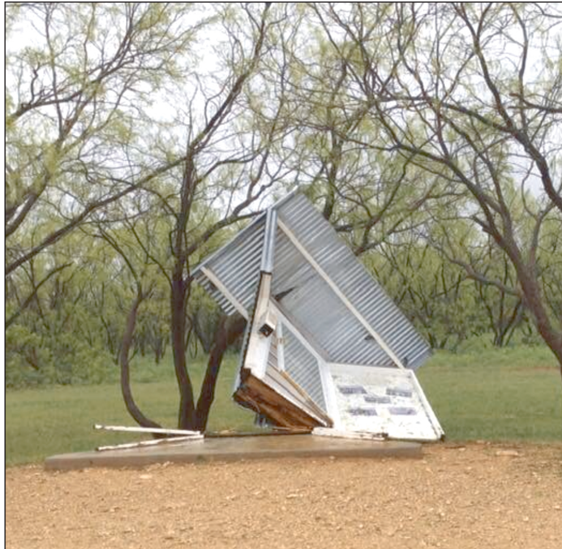
Storm Damage! This information kiosk at Fort Chadbourne was one of the things damaged due to the storms that rolled through the area Tuesday evening, April 23, 2019. Some residents of Oak Creek Lake also experienced power outages from downed lines and snapped poles from the storm, as well as hail damage.
