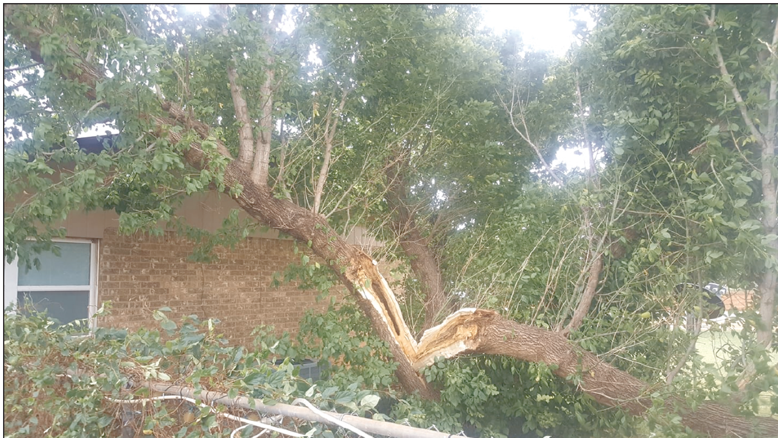
High Winds! Friday evening, June 23, 2017, thunderstorms with lots of lightning and extremely high winds swept through Coke County. Numerous trees and roofs were damaged. However, the county dodged a bullet which might have rivaled the Wildcat Fire of 2011. Lightning set numerous fires which were extinguished, but a fire in the Poverty Canyon area southwest of Tennyson was the one with which officials were concerned. Poverty Canyon residents were evacuated and both Bronte Volunteer Fire Department and Robert Lee Volunteer Fire Department, along with other area agencies and departments, battled the blaze. Thanks to divine providence and dedication by the first responders, the fire was contained.
