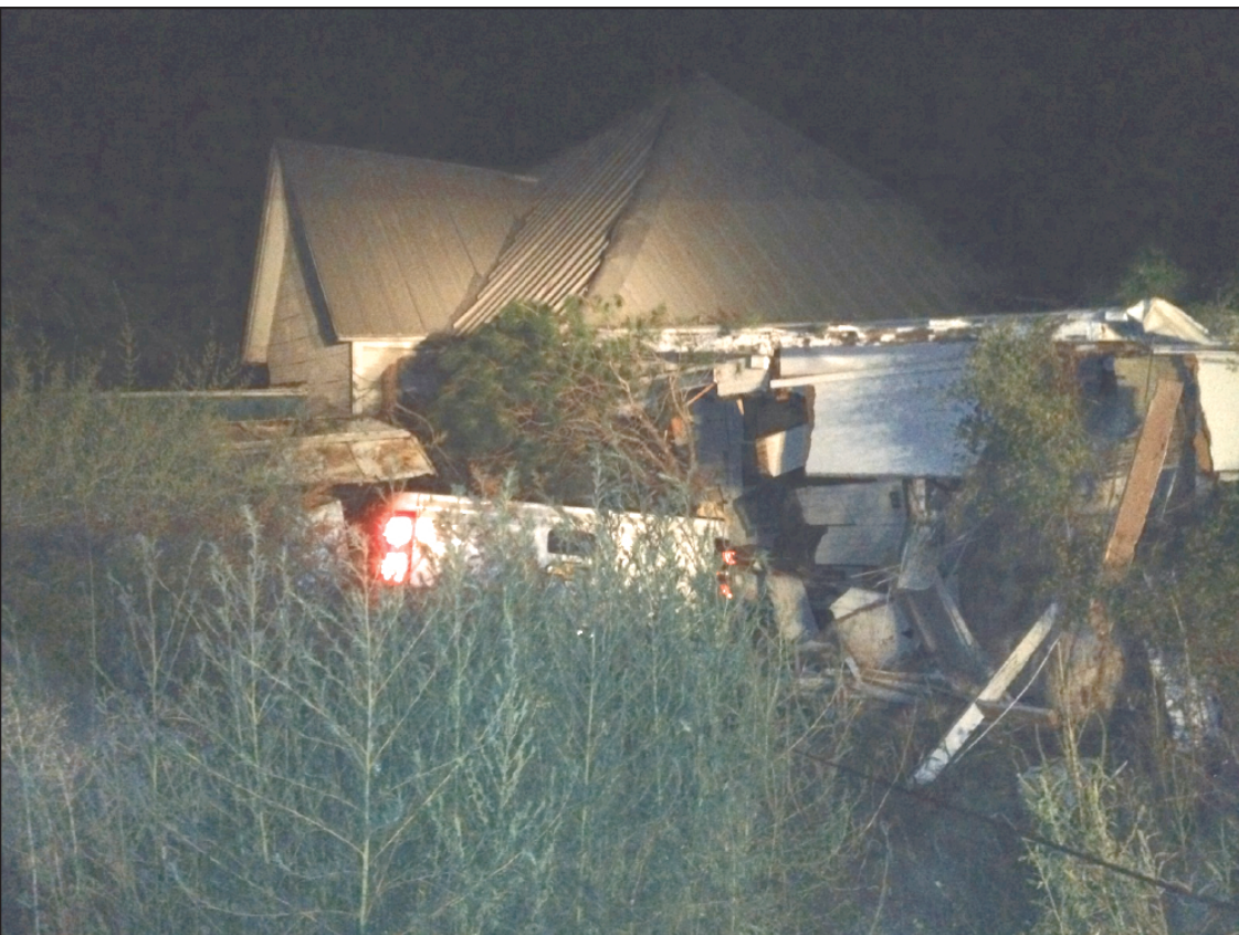
House Damaged! At approximately 2:40 am Saturday morning, July 25, 2015, a pickup crashed into the home at 1010 Austin Street in Robert Lee. The driver of the pickup is from Snyder and while traveling northbound on State Highway 208, failed to negotiate the curve on State Highway 208 just past the State Highway 158 intersection. The driver was arrested for driving while intoxicated by DPS Trooper Dykstra. Also assisting with the accident were Coke County Chief Deputy Brandon Neal and Deputy Terry Crenshaw. A resident of the home was taken by ambulance to the hospital, but was treated and released.
