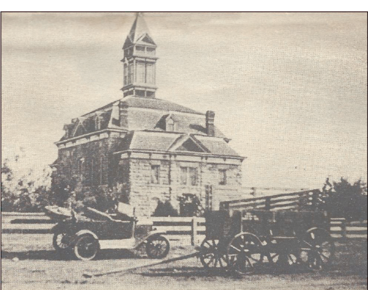
Coke County Courthouse! In the spring of 1891, the cornerstone was laid for the new Courthouse that was to be the home of Coke County's government for the next 65 years. Built of native stone quarried by hand, most of the stone came from the Kirkland Ranch and hauled to Robert Lee in wagons.
