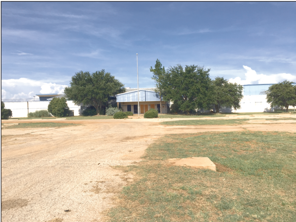
Old Coke County Detention Center
